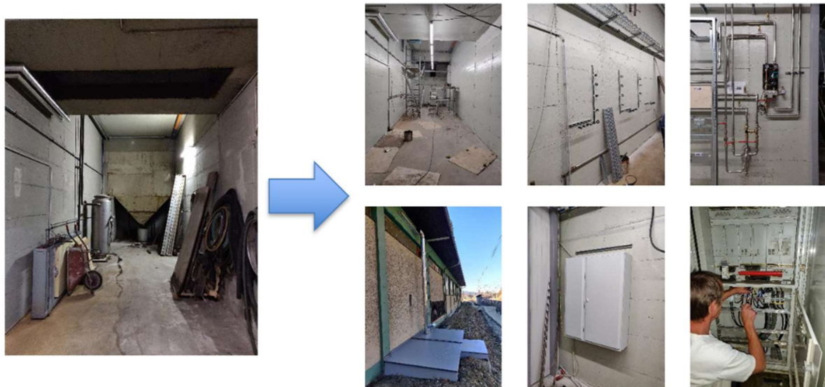
Figure 29. Preparation of the technical room for installation
