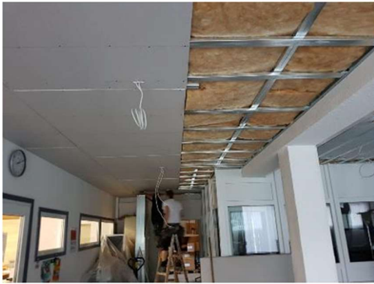
Figure 32. Cooling/heating ceiling installation
