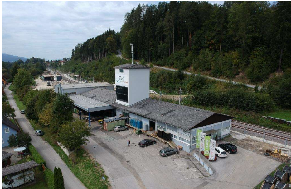
Figure 28. Langenwang demo building
