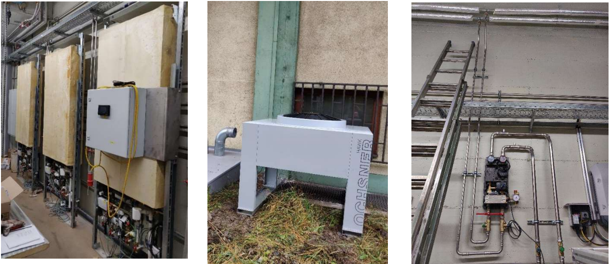
Figure 31. PINK storage, hydraulic network and, Ochsner outdoor unit installation
