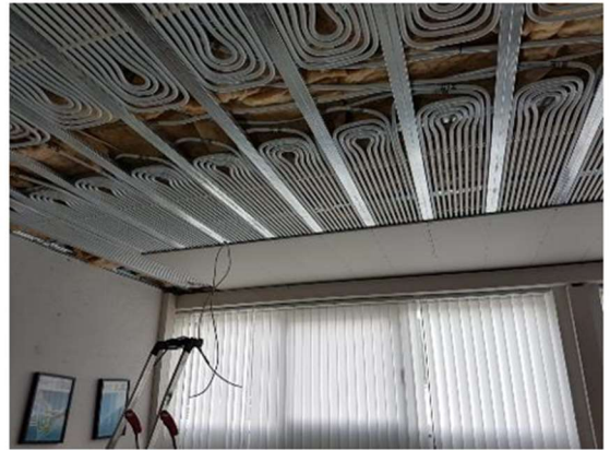
Figure 32. Cooling/heating ceiling installation
