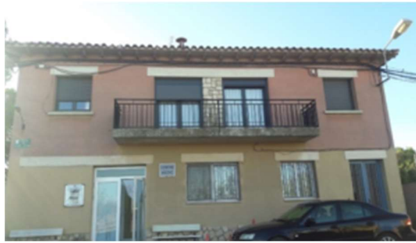
Figure 3. Almatret demo site building
