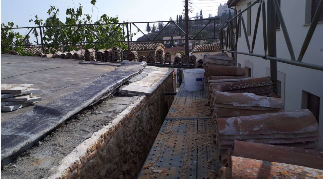
Figure 15: Photo from the installation of roof insulation
