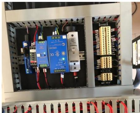
Figure 18: devices for storage control integrated in the rack.
