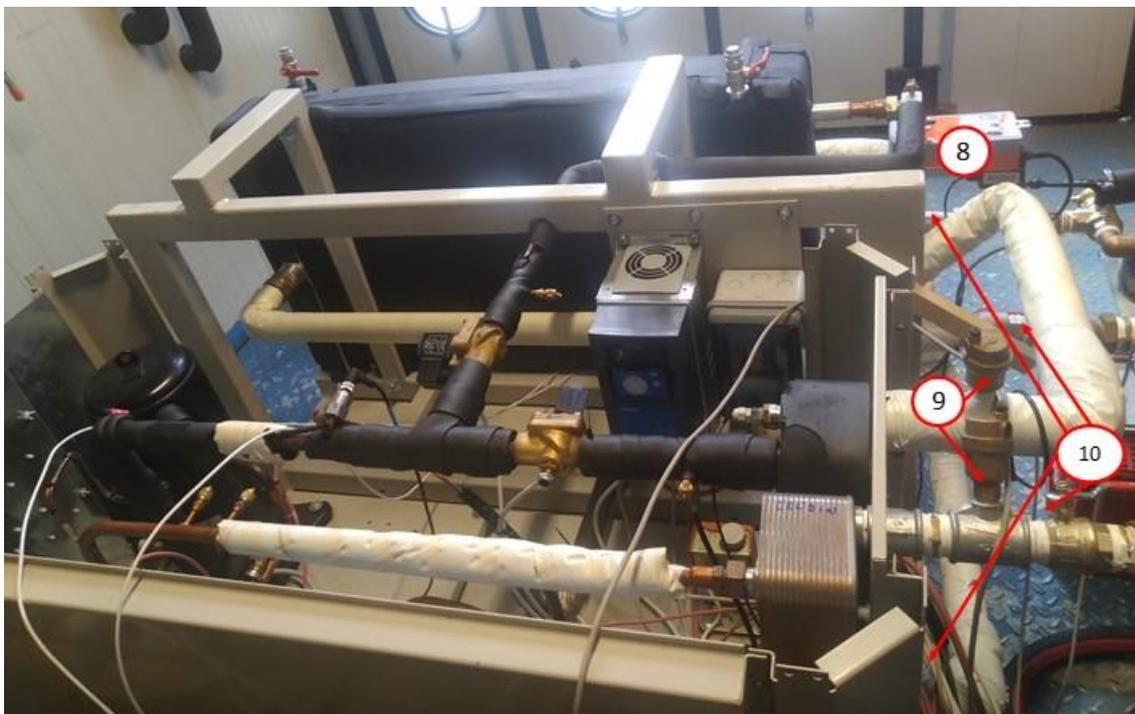
Figure 7: integration of the latent thermal storage in the heat pump – focus on hydraulic circuit. 8: 3-way valve, 9: air traps, 10: manual ball valves.
