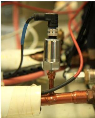
Figure 10 Pressure and temperature sensors in the refrigerant circuit
