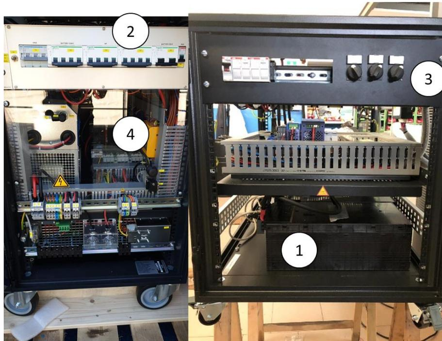
Figure 17: integration of DC bus and electric storage. 1: batteries; 2: main switches; 3: manual switches; 4: main PLC.
