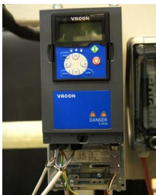
Figure 12 The DC-driven VACON inverter (Variable Speed Drive) of the compressor
