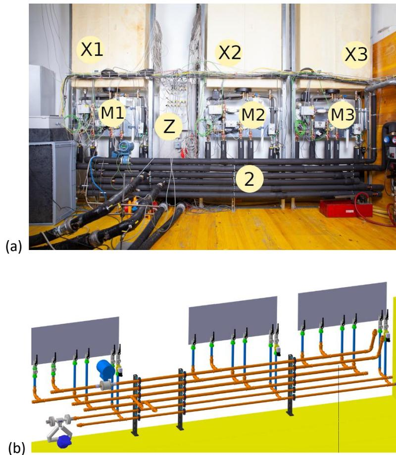
Figure 32: Connections and piping. (a) Photo of the hydraulic connections. (M1)-(M3) hydraulic modules, (X1)-(X3) 140 liter DHW enerboxx storages, (Z) B&R DAQ, (2) connecting pipes. (b) CAD drawing of the piping
