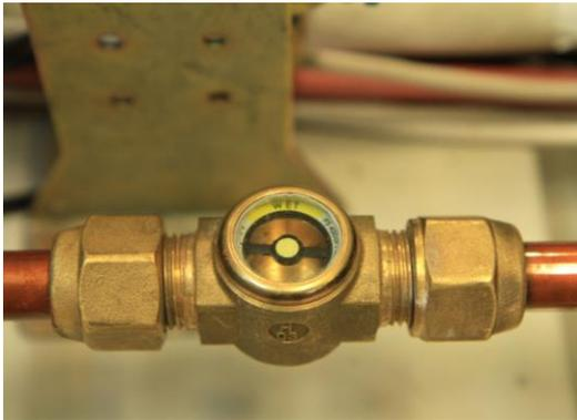
Figure 8 Sight Glass in the refrigerant circuit
