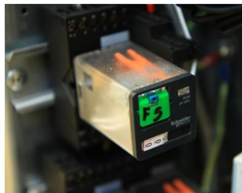
Figure 13 The by-pass relay of the Flow Switch
