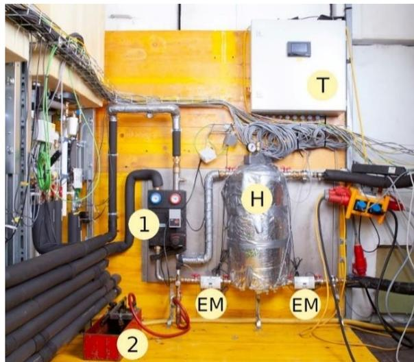
Figure 34: Interface between HP internal and building water cycle. (1) water pump (K in Figure 23), three-way valve (U in Figure 23) and temperature sensors integrated in a compact box, (2) filling station for the process water, (EM) energy meters, (H) hydraulic separator (Please note that the uninsulated hydraulic separator can also be seen in Figure 30b), (T) thermal controller.
