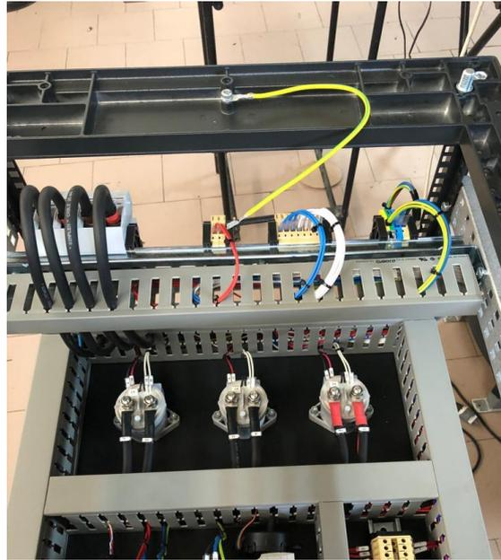
Figure 19: power breakers and safety disconnection coil.
