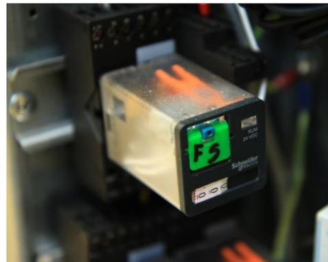
Figure 13 The by-pass relay of the Flow Switch
