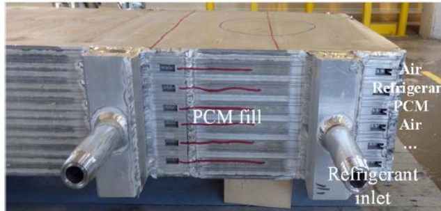
Figure 1. Photo of the heat exchanger for refrigeration dryer with integrated PCM storage.
